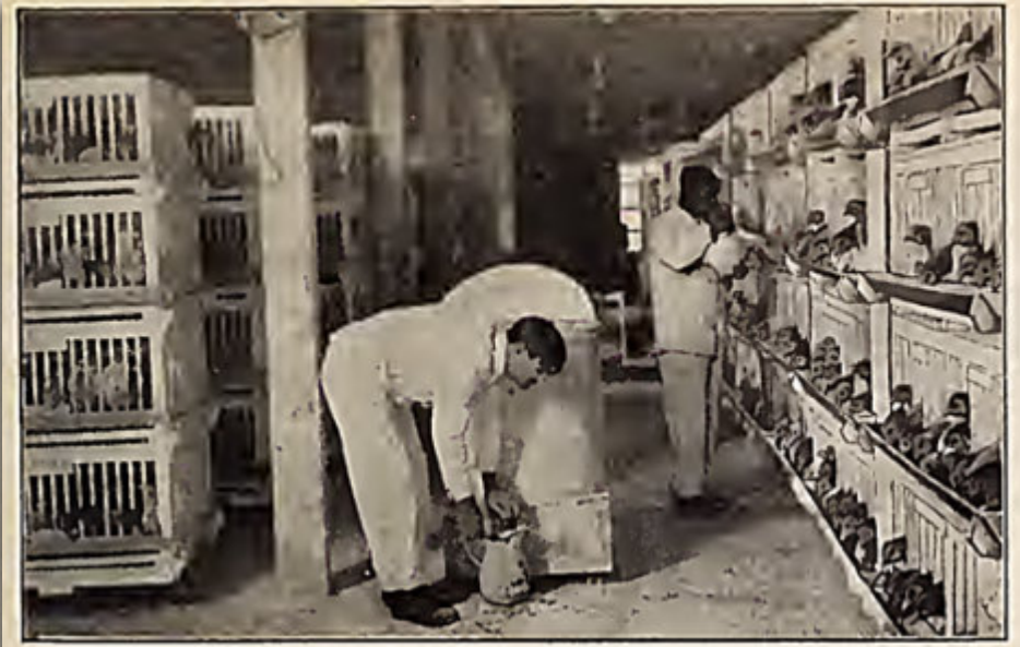
The Naive-Spillers company's plant has a fattening capacity of 10,000 chickens every two weeks. Above is shown a sectrion of the feeding 'batteries' where the purchased chicks are cooped and fed special rations, in which sour milk plays an important part. The feed mixer is on wheels (behind the man with the jug) so that it can be pushed about for convenience. Below: A manure truck at the large milk-feeding plant.
